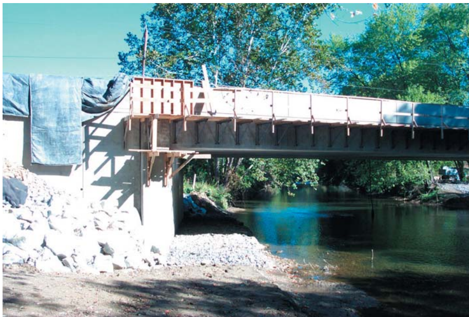
State Route 151 Bridge Over Raccoon Creek - After
