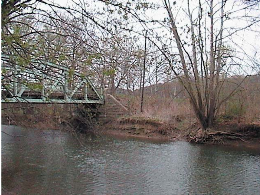
State Route 151 Bridge Over Raccoon Creek - Before
