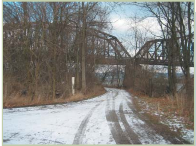
Bridgewater Crossing - Existing CSX Bridge Underpass
